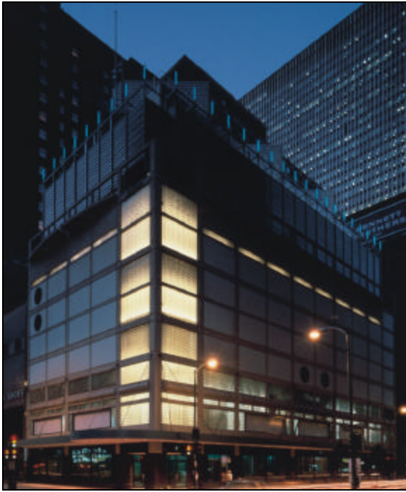
Unicom Thermal's flagship refrigeration plant in the heart of downtown Chicago.
