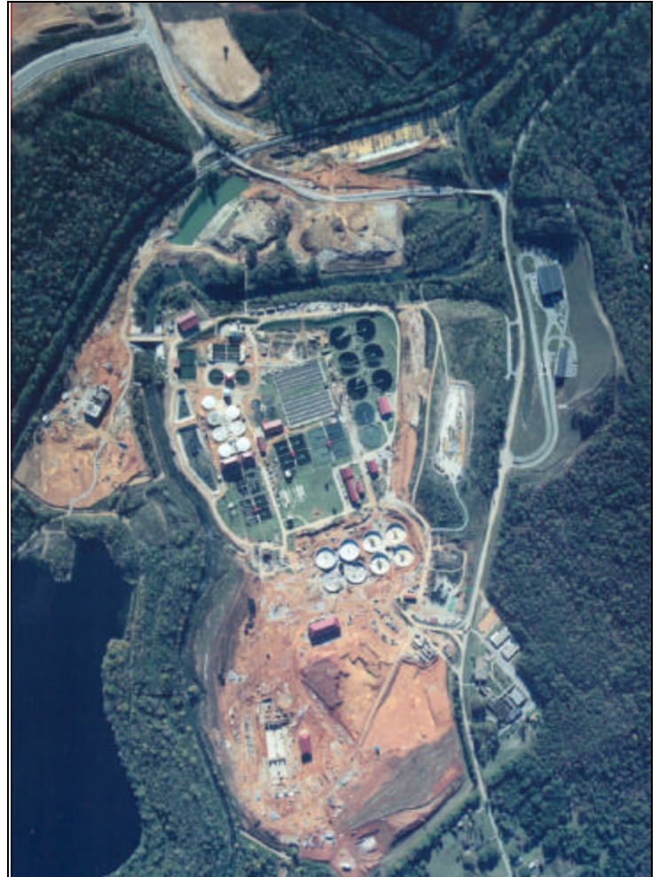
Seen here is an aerial view of the huge Valley Creek Waste Water Treatment Plant in Bessemer, Alabama.
